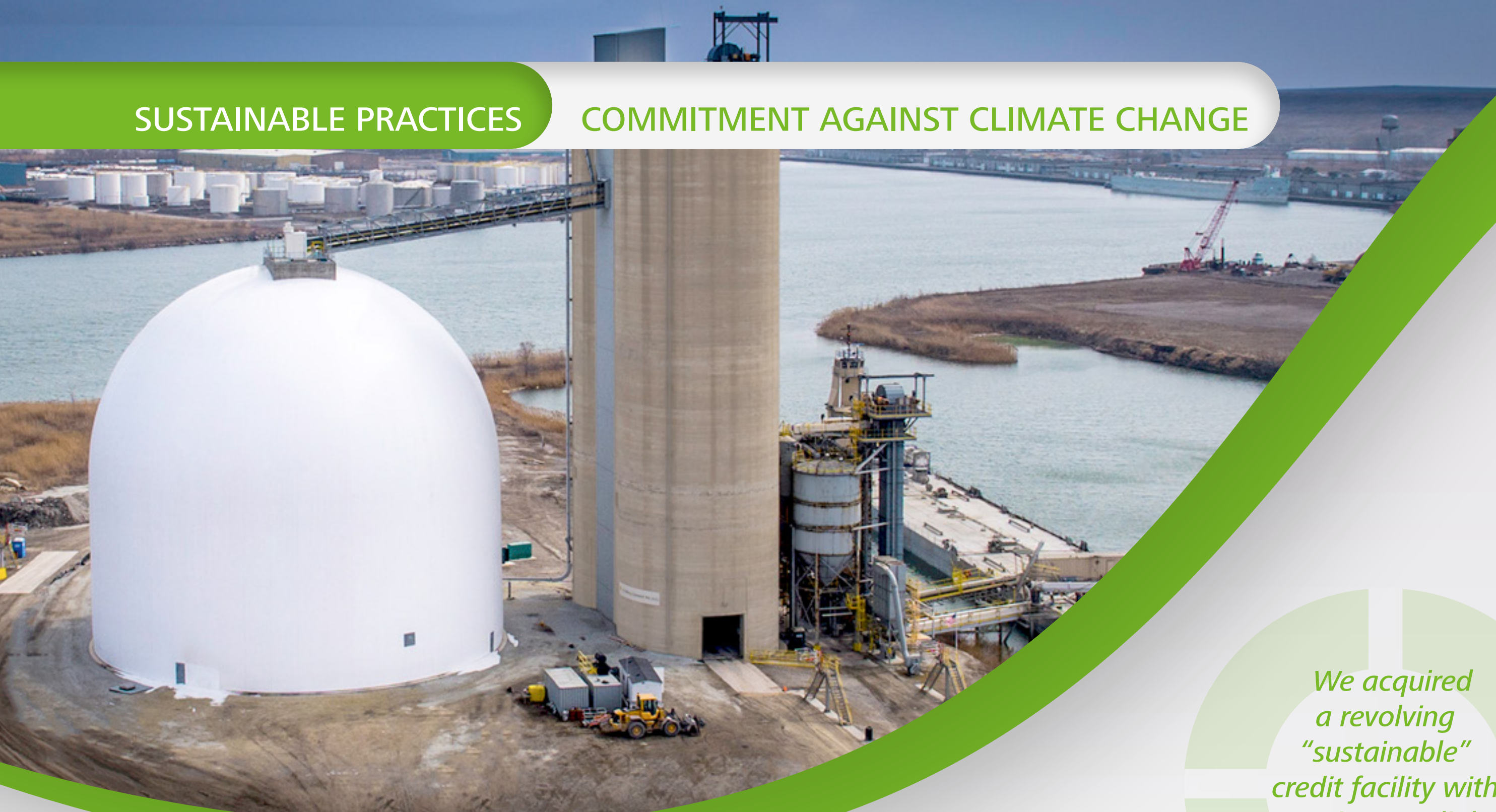
Chicago Terminal in USA
